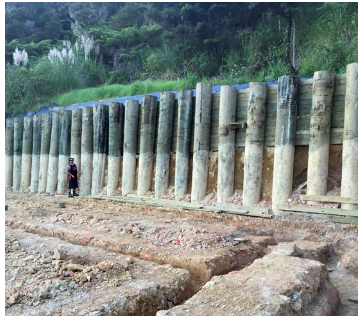
Photos courtesy of Markovina Pile Driving
